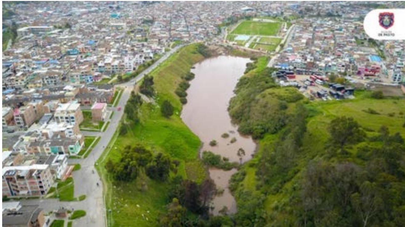
Fig. 12: Landslide emergency in Guachucal Stream Source: Majority of Pasto, 2024
